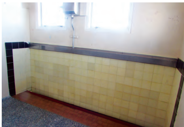
The Men's toilets at the Kapuni War Memorial Hall are in need of an upgrade.
